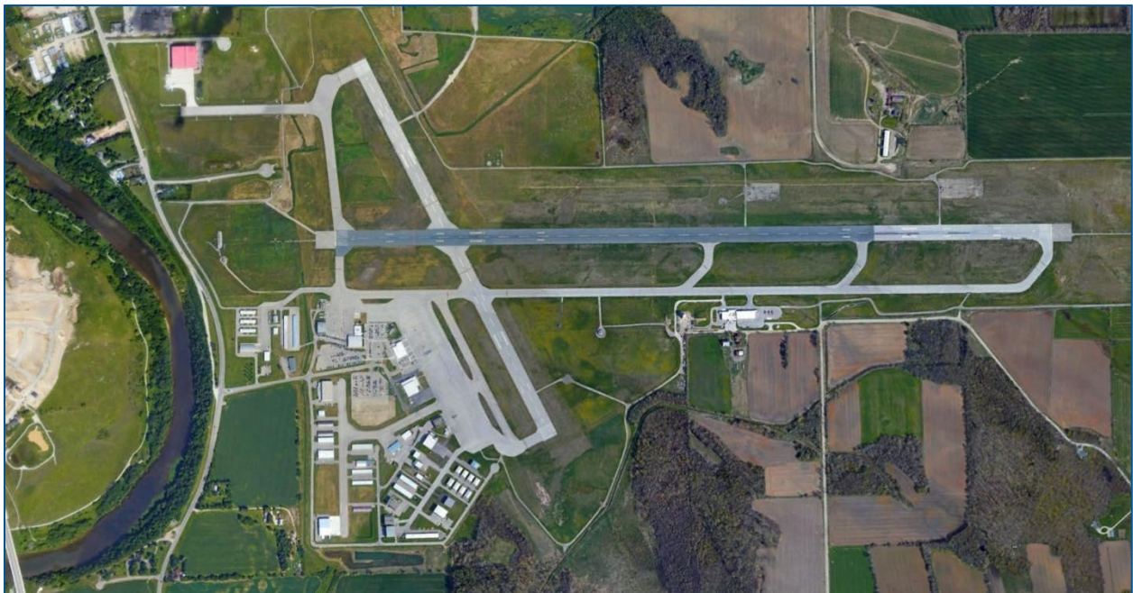
Region of Waterloo International Airport
