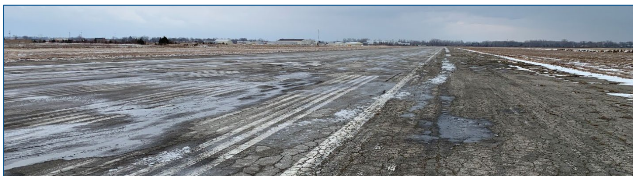
Secondary runway at Sarnia Chris Hadfield Airport
